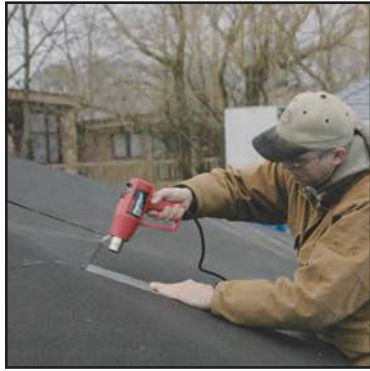
Weld Roofing Membrane
