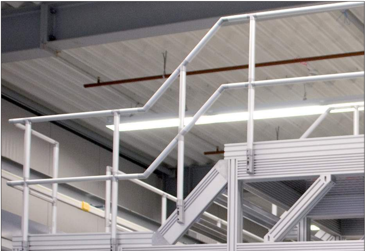
Staircase between two operating platforms.
