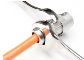
Step 17 - Tighten to 5-7 N/M using 25mm wrench
