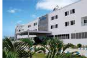
Rudrapur Plant (Green Building)
