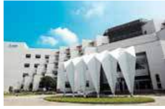
Tainan Plant (Diamond-rated Green Building)
