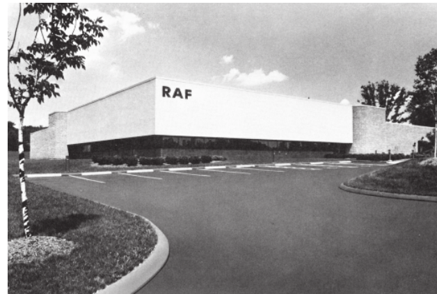
U.S. manufacturing and plating facility
