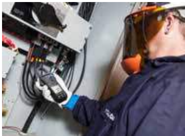
Analyze Power-related Issues
