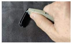
14. Use a utility knife to open the bottom of the grommet to accommodate the patch cables.
