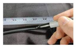
4. Measure 27-inches from the end of the cable an make a mark with a black marker. Feed the grommet over the cable beyond the mark on the cable jacket.
