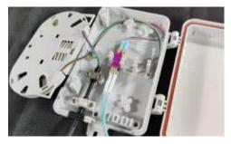
13. Plug the connectors from the distribution cable into the appropriate fiber optic coupler. Any unused fibers can be routed to the side the box for future use. Reinstall the cable "T" at the top end of the distribution box.
