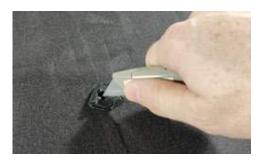
3. Remove the cable grommet with the large opening from the distribution box. Use a utility knife to cut the scored "X" to help pass the cable into the box.
