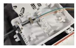
7. Reinstall the cable clamps for the distribution cable and verify the cable is secure.
