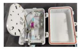
16. Reinstall the cable clamp for the patch cables. Carefully Reinstall the splice tray in the hinge locations.
