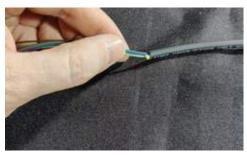
5. Remove the jacket at the mark and cut off the aramid fiber.
