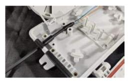
6. Wrap electrical tape around the cable where the cable clamps are located to ensure a secure fit. Make sure the grommet is fit into the body of the distribution box.
