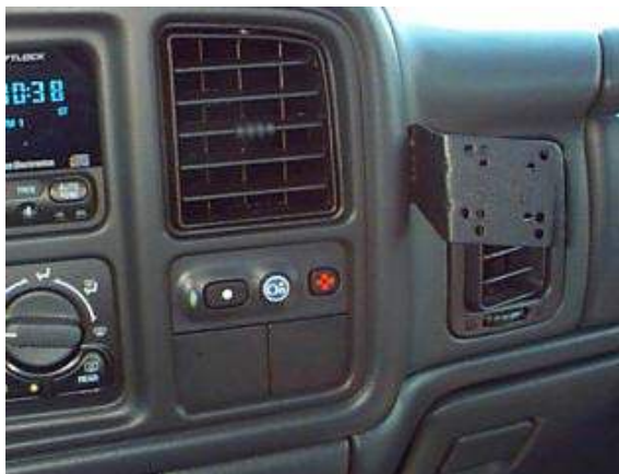
Finished Installation Picture
