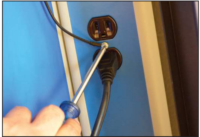
Figure 8B. Grounding the SCS 724 Workstation Monitor
