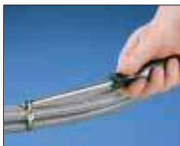
Installer controlled tension.
