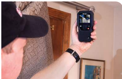
Scanning ceiling & wall joint for moisture issues
