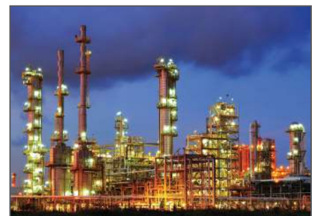
Oil and gas, chemical and petrochemical Plants
