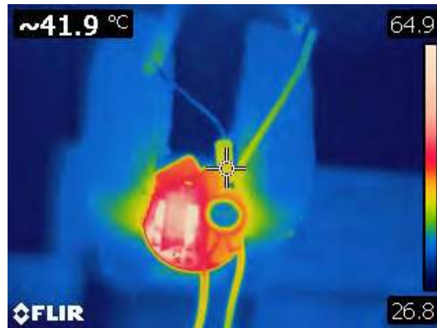
Figure 37 – 300 VAC, 48 V LED Load. Spot 1: Fusible Resistor (RF1): 41.9 °C.
