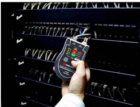
Confirm continuity and fault type
