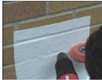
Using TSA-2 to work film into mortar joints
