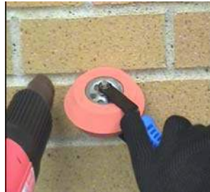
Using TSA-2 to work film into mortar joints
