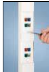
Install faceplate over module frame.
