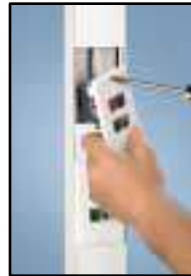
Screw module frame and faceplate together.
