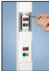
Terminate jacks, snap jacks into module frame and screw module frame to faceplate bracket.
