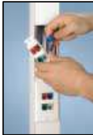
Terminate jacks and snap into module frame.
