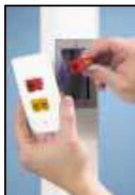
Terminate jacks and snap jacks into faceplate.
