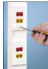
Install faceplate over bracket.
