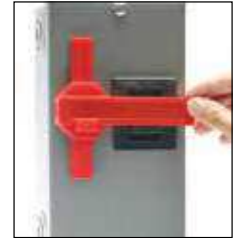
Slide Stop Bar into position over breaker
