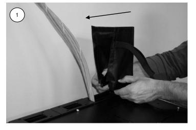
Step 1: Disengage the hook and loop cinch tie and the hook and loop strips along the top edge and side of the fabric sleeve. Open the fitting to accept the existing cable bundle by separating the end of the fitting assembly.
