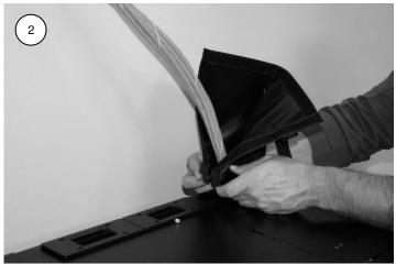
Step 2: Place the fitting around the cable bundle.
