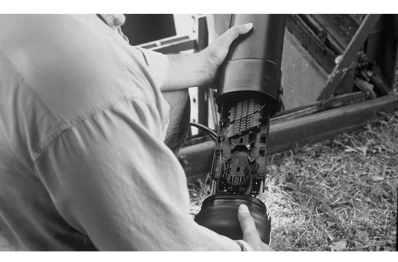
3M Dome Splice Closure FD protects fiber optic splices from the elements while providing fast and easy no-cost reentry. These closures can be installed in above-ground pedestals, hand-holes, and mounted on poles and strands. The closure utilizes proven sealing technology and over 30 years of experience with copper protection.
