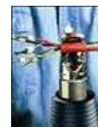
Applying Shrink Tubes
