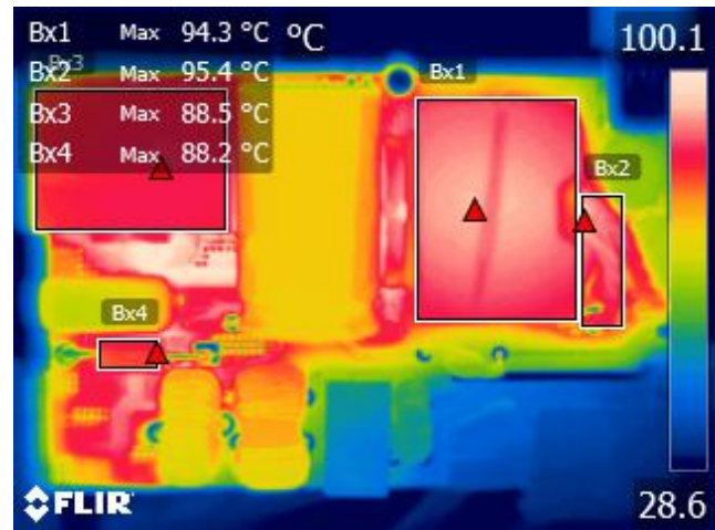
Figure 59 – Top Thermal Image, T_{AMB} = 27.9 °C. Bx1: Transformer Core = 94.3 °C. Bx2: Transformer Wire = 95.4 °C. Bx3: PFC Inductor Core = 88.5 °C. Bx4: Boost Pre-charge Diode = 88.2 °C.
