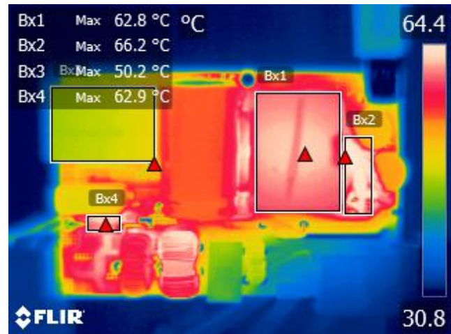
Figure 47 – Top Thermal Image, T_{AMB} = 28.3\text{ }^{\circ}\text{C} . Bx1: Transformer Core = 62.8 °C. Bx2: Transformer Wire = 66.2 °C. Bx3: PFC Inductor Core = 50.2 °C. Bx4: Boost Pre-charge Diode = 62.9 °C.
