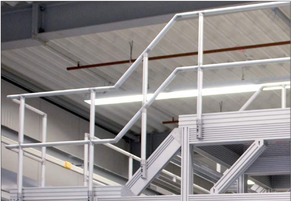
Staircase between two operating platforms.
