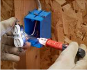
Test wires for AC voltage
