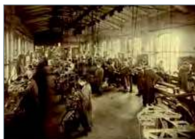
Montage und Mechanikfertigung in Göttingen um 1910 Mounting and mechanics production in Goettingen about 1910
