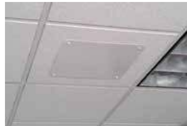
Installed Condition: PSIBVHF and PSIBVU78
