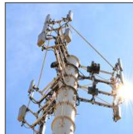
Cellular Base Station
