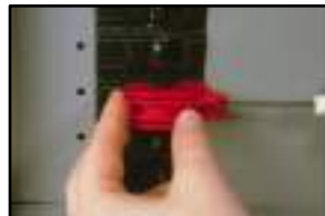
Tighten set screw securely with standard screwdriver.
