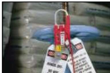
Gate Valve Lockout Device
