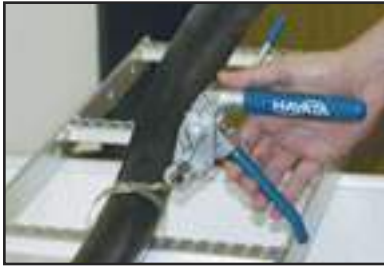
Place band in position and hand tighten as much as possible.
