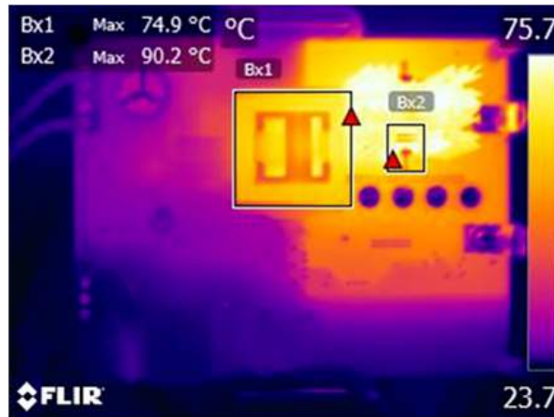
Figure 15. Thermal Image Top
