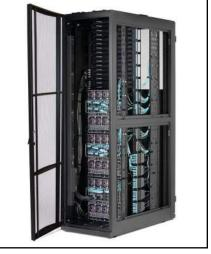
Belden Zero U - Vertical patch panel allows for optimal use of mounting space into XS Series enclosures by providing high-density connectivity options along the equipment mounting rails.
