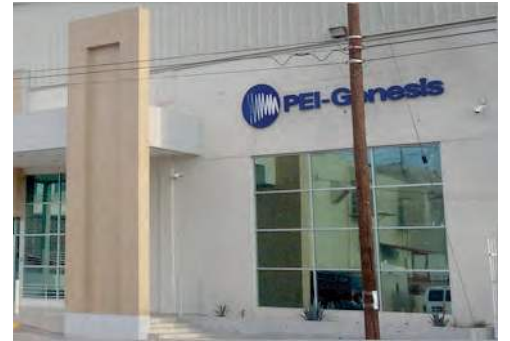
Production Facility, Nogales, MX
