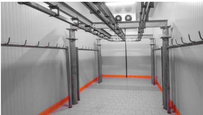
Cold Room and Storage
