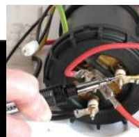
Water Heater Installation
