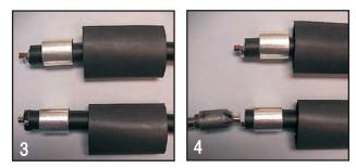
**Step 3:** Lightly score the circumference of the cable 0.20" back from the end of the core. Make one long longitudinal cut. Pry up a piece of the jacket and gently peel the ring of the jacket off the core.
