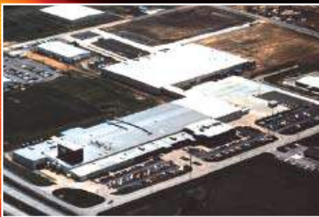
The EnerSys® plant in Warrensburg, Missouri covers 32,000 square feet and is situated on 33 acres.
