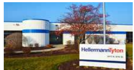
Offices and Manufacturing 87th Street, Milwaukee, WI
