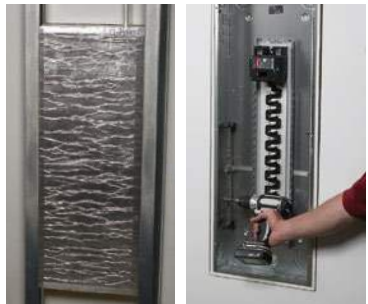
High-performance endothermic mat with protective aluminum foil.
