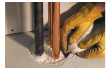
3M™ Fire Barrier Packing Material PM4 is approved for use in all 3M through penetration firestop systems requiring backing material.
