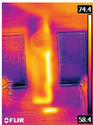
Warm Drain Pipe in Wall
