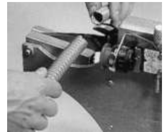
The result is a clean and finished cut of the conduit
