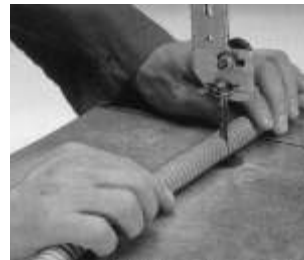
Lightly cut through conduit
