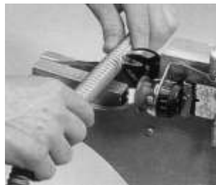
Cut into the plastic sheathing
