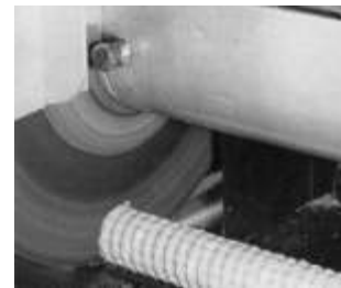
Lightly cut through the conduit for clean ends.
