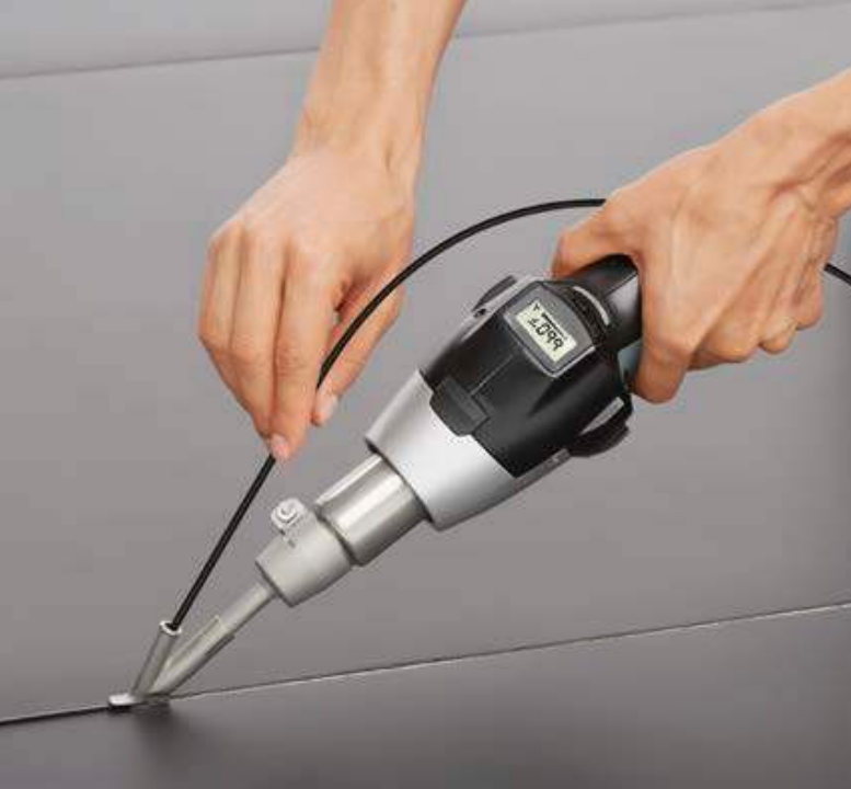
▲ Welding linoleum HG 2620 E
