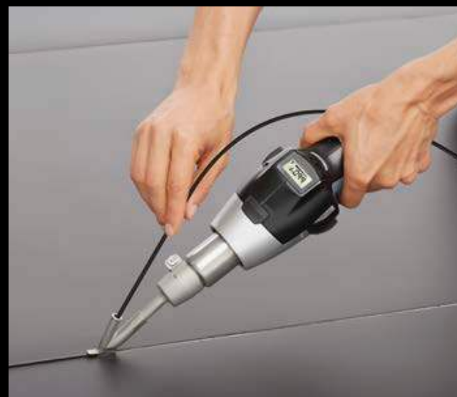
Welding linoleum floors.
