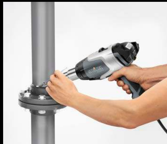
Welding plastic in tank and apparatus construction.
