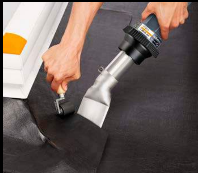
Overlap welding on a light dome.
