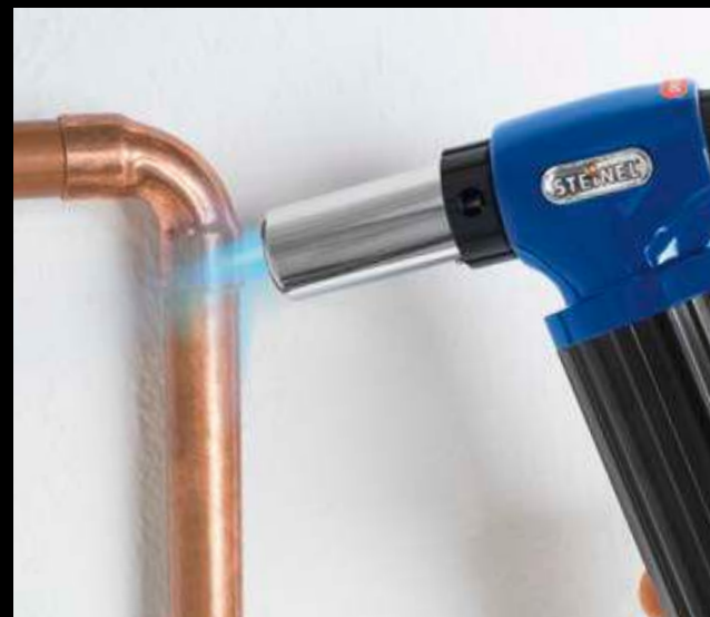
Solder joints on copper piping
