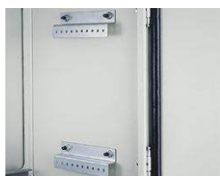
Perforated rails installed on lateral studs.
