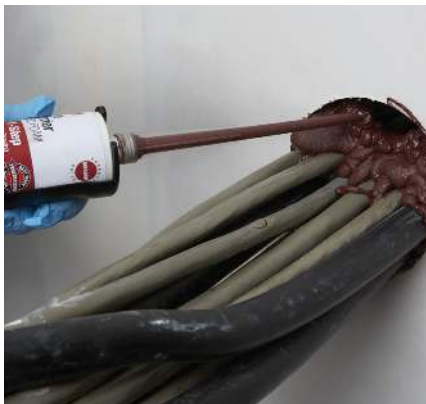
Firestop HVAC line sets: 3M™ Fire Barrier Rated Foam FIP 1-Step ( pg 33 )
