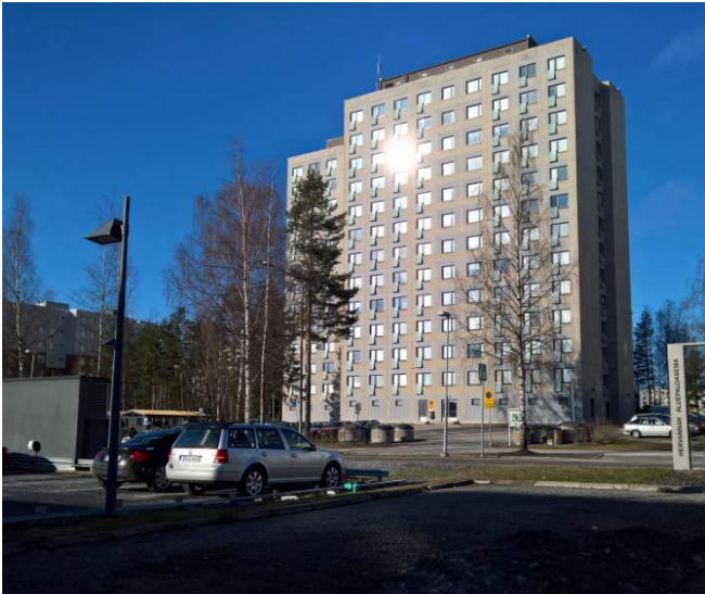
Base antenna 4 on silver car, looking west
