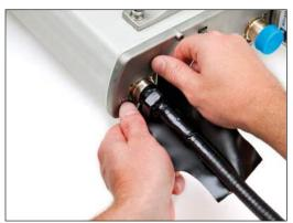
3.4 Starting 1" below the butyl mastic tape, wrap one half-lapped layer of 2" (51 mm) vinyl tape up to the base of the antenna. Repeat the procedure to apply second half-lapped layer.
