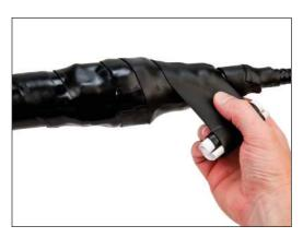
2.6 Next, beginning 1" (25 mm) beyond the layer of butyl mastic tape applied in step 2.5, wrap the entire section of cable with one or two layers of half-lapped 2" (51 mm) wide vinyl tape extending 1" (25 mm) beyond the layer of butyl mastic tape.
