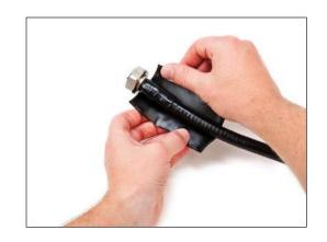
4.3 Starting 1" (25 mm) below the butyl mastic tape, wrap one half-lapped layer of 2" (51 mm) vinyl tape up to the connector clamping nut. Repeat procedure to apply second half-lapped layer.
