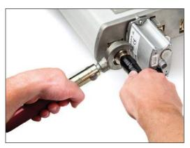
4.6 Start 1" (25 mm) below the connector clamping nut and apply one (1) halflapped layer of <sup>3</sup>/<sub>4</sub>" (19 mm) vinyl tape extending 1" (25 mm) beyond the cable connector clamping nut. Wrap up to, but short of, the base of the antenna. If space restrictions prevent wrapping tape from roll, then the tape can be applied in one (1) or more strips if necessary, or a strip can be wound onto a small applicator, (e.g. a pencil), and unwound around the connection assembly.
