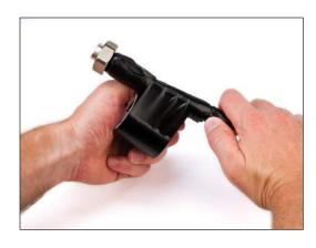
4.4 Starting 1" (25 mm) below the previous vinyl tape layer, wrap the cable with three continuous half-lapped layers of ¾" (19 mm) wide 3M™ Scotch® Super 33+™ Vinyl Electrical Tape up to the connector clamping nut.
