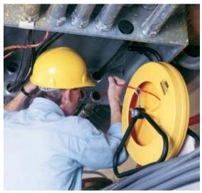
Lightweight, portable unit typically used for running inside and outside conduit drops as well as home drops from the hand-hole box to a building. Also used for light pole and control wiring or walker ducts.
