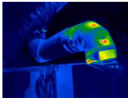
INSPECT DUCTS AND VENTILATION
