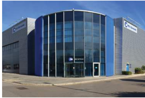
European Headquarters & Production Facility, Southampton, UK
