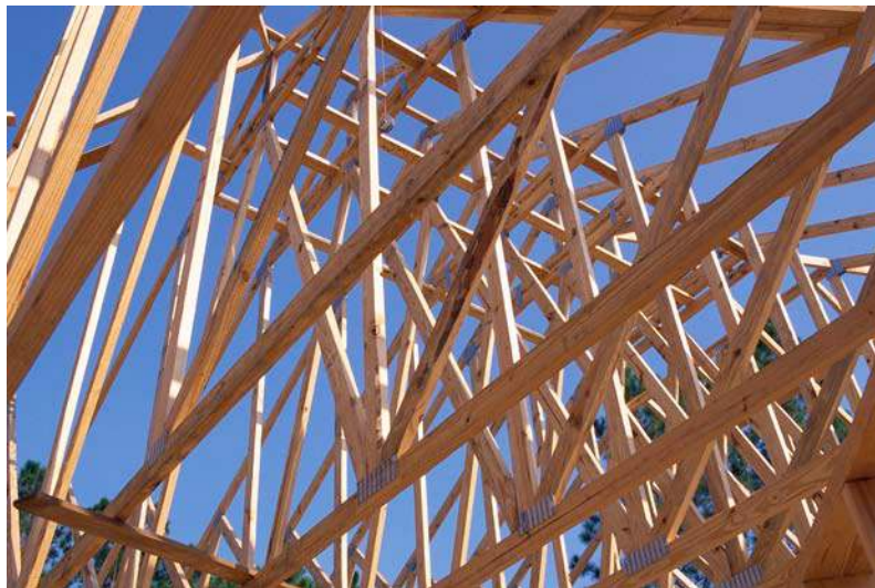
Photo 1. With fiber optics being used more and more, some new home builders are installing fiber optics during construction.
