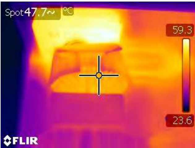
Figure 71 – Differential Mode Choke (L4), 230 VAC Input, 100% Load, Room Temperature.
