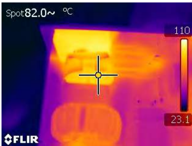
Figure 51 – Differential Mode Choke (L4), 90 VAC Input, 100% Load, Room Temperature.
