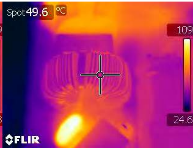
Figure 60 – Common Mode Choke (L1), 115 VAC Input, 100% Load, Room Temperature.
