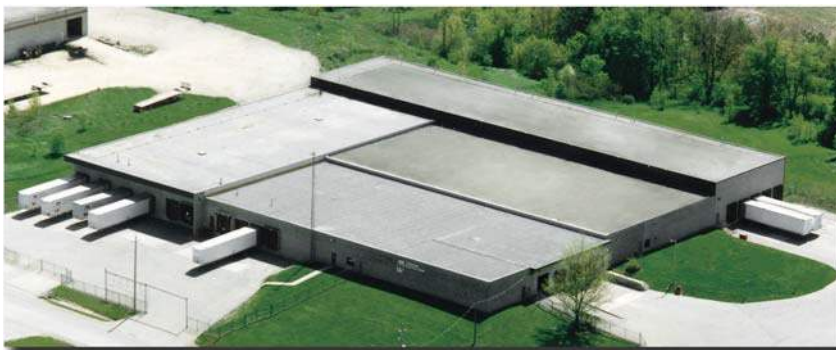
Hammond North American Distribution Centre
